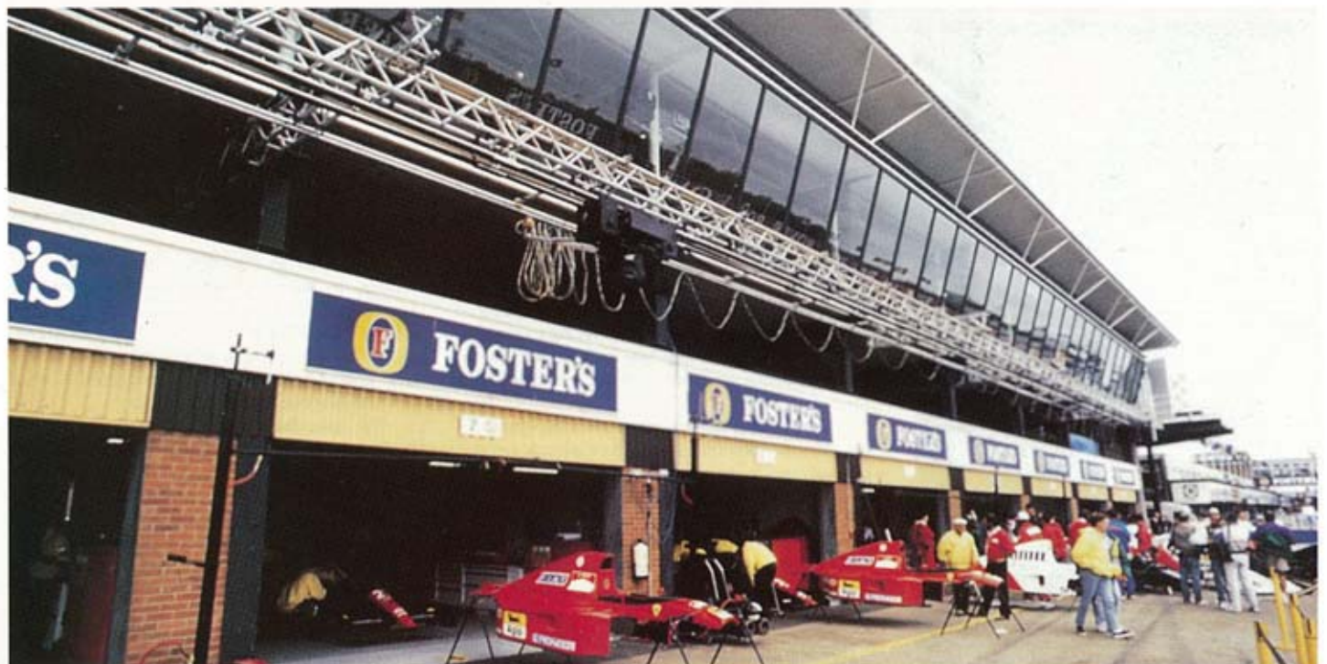
Camtrak at Silverstone: the 'over pit' view is provided by cameras tracking on the cantilevered system.
