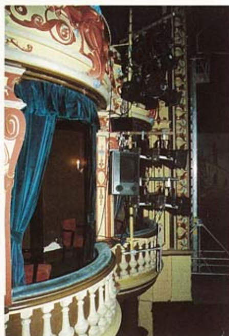
Close-up of flown 'Force 9' part of the Ambisonic set-up at the Theatre Royal in York.
