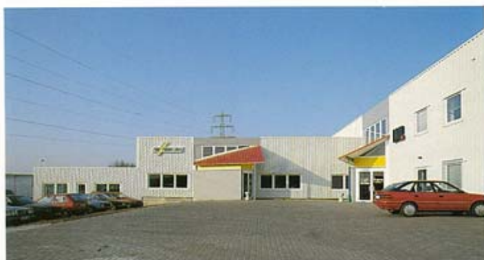
LMP Lichttechnik's impressive facility.
