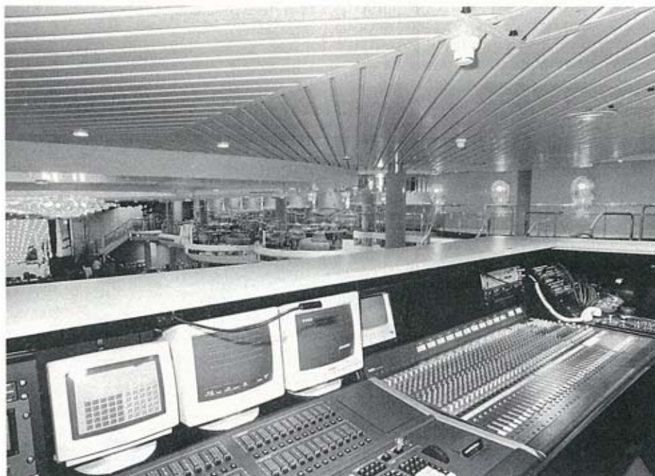
Show lounge controls. Light Palette 90 and Yamaha PM 1800s side-by-side in the control point which has moved to the back of the auditorium.
