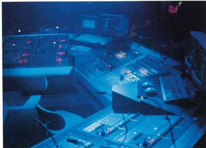
The light control booth with 16 computers controlling 11 separate lighting systems including Time Code shows.
