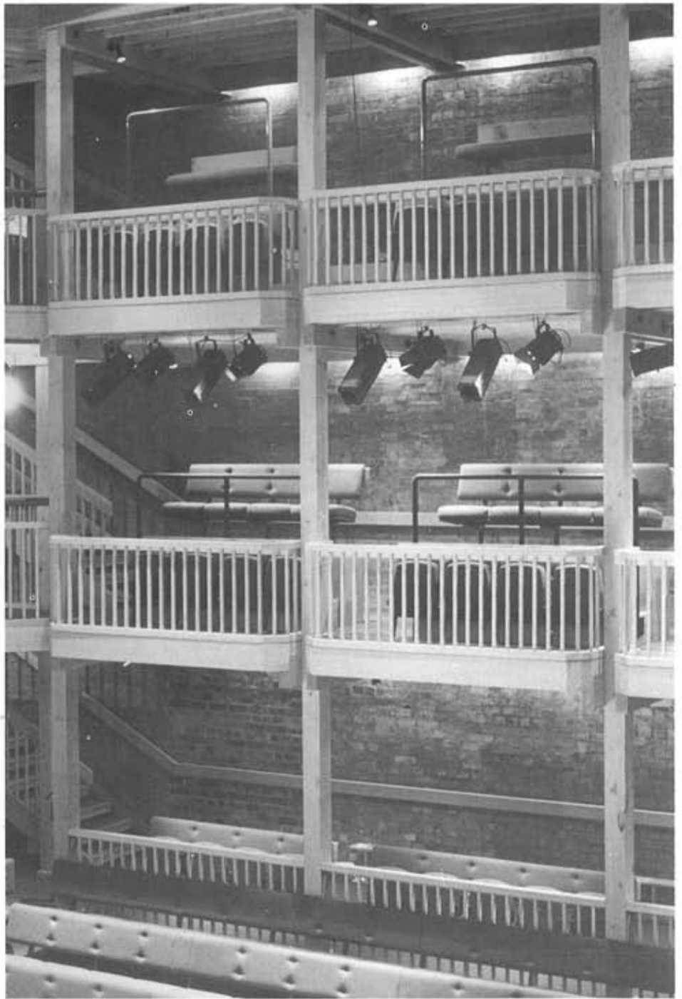
Spectator galleries with lighting bars suspended underneath.
