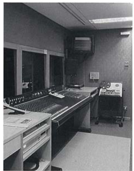
The sound control room with Soundcraft desk and Revox tape machine.
