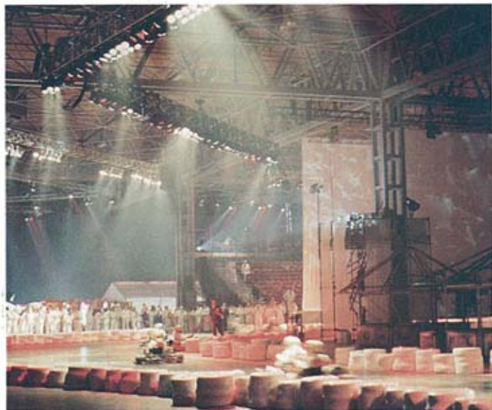
The karting track was lit with over a 1,000 Parcans, and a cluster of molefays, molemags and lekos.
