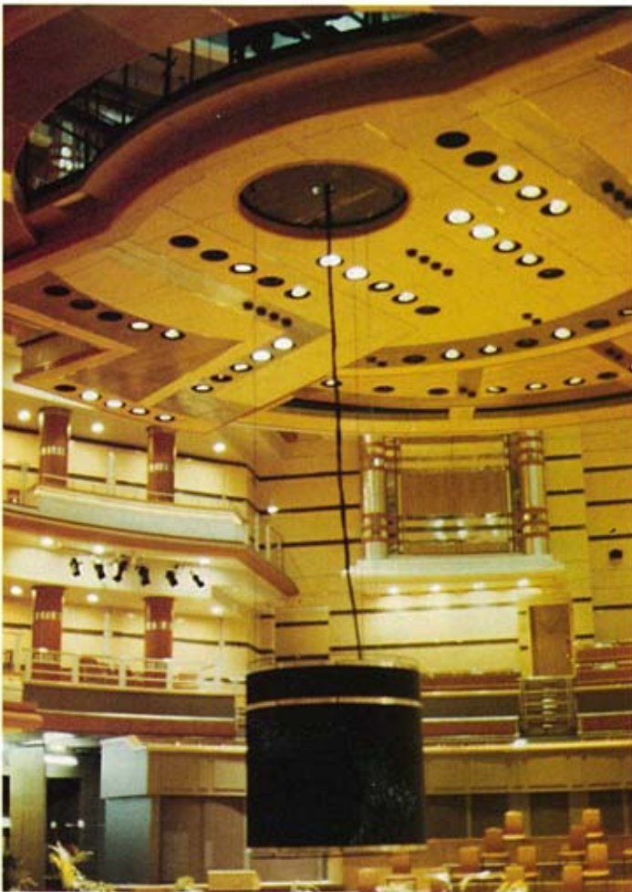
Symphony Hall: the central speech cluster lowered from the acoustic canopy above.
