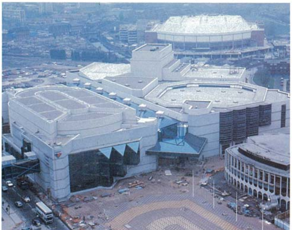
The new Birmingham International Convention Centre with Indoor Arena in background, and Symphony Hall to the left. The existing Birmingham Repertory Theatre is in the foreground, right.
