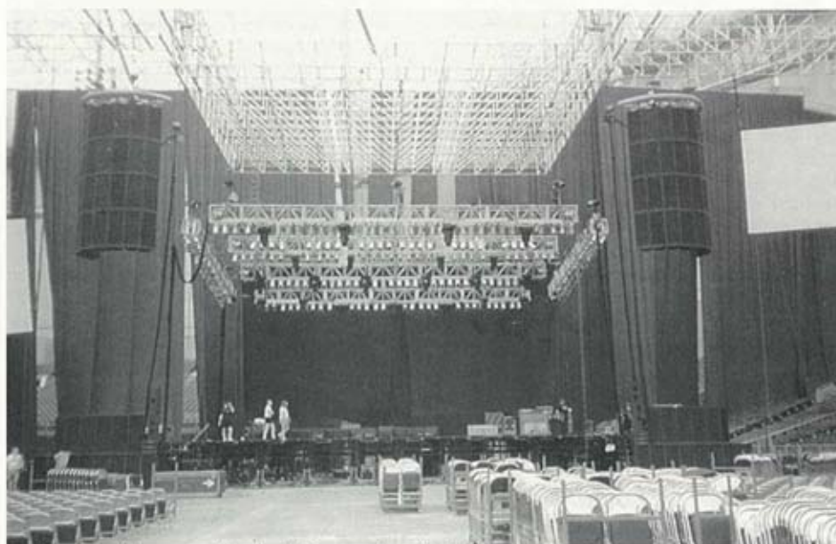
The box rig with staggered, split single trusses installed in the St. Petersburg Arena in the States.
