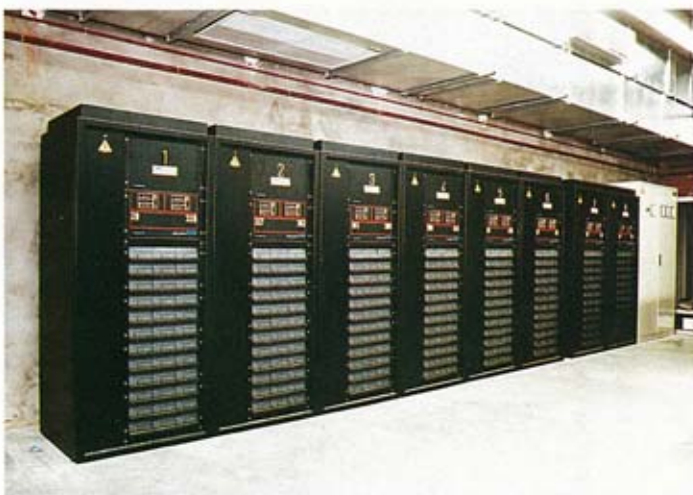
Eurodim digital dimmers at RTBF in Brussels.
