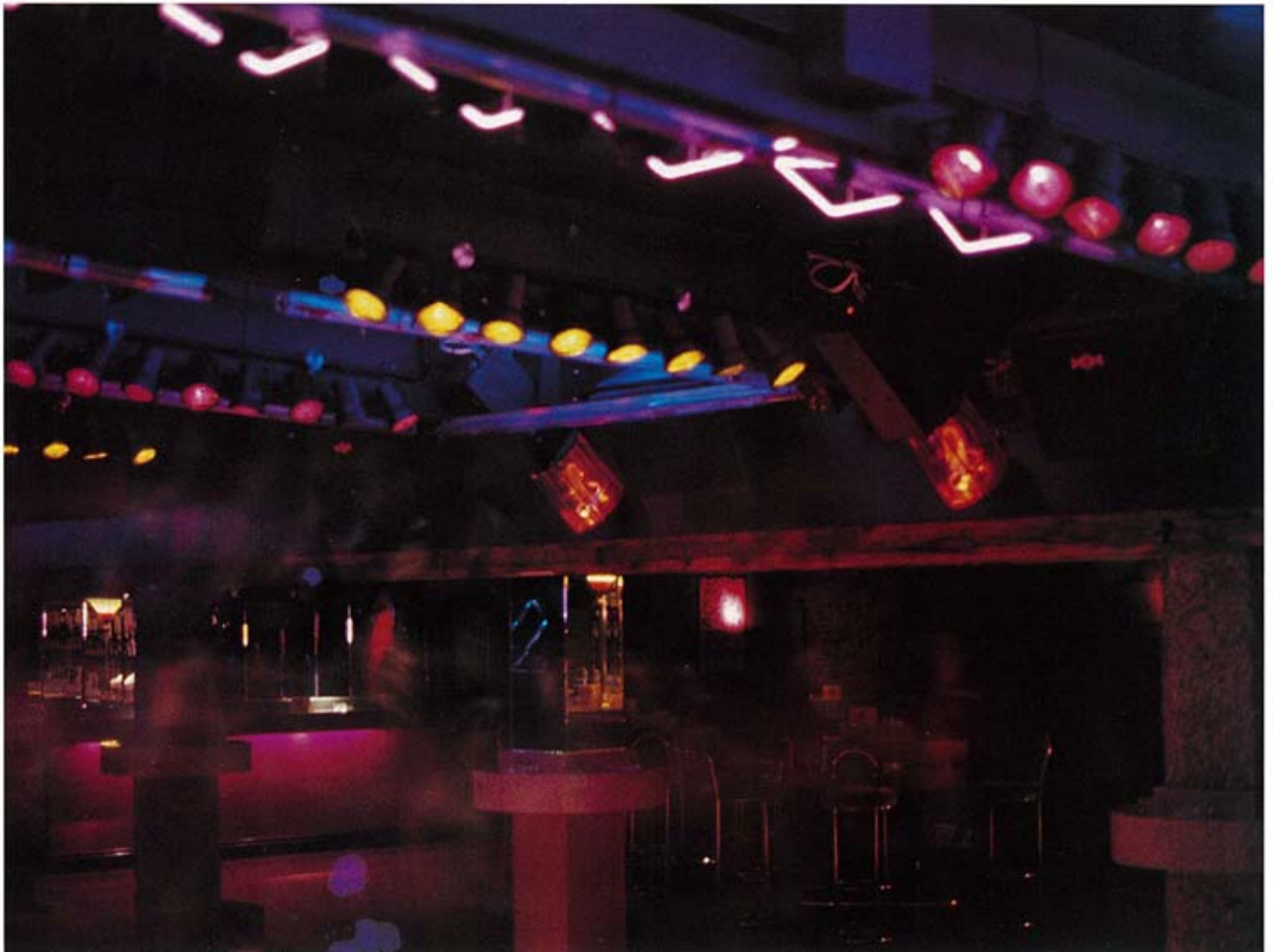
The Barn: Laser Systems' Colour Sweeps can be clearly seen in the centre with neon chasing effects above.
