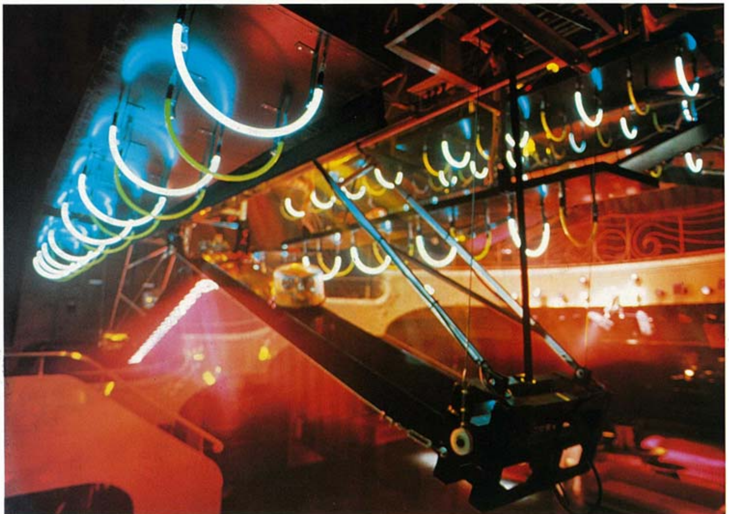
A close view of one of the rigs showing the light curtain. The neon flaps fold down to form a tunnelled neon ceiling.
