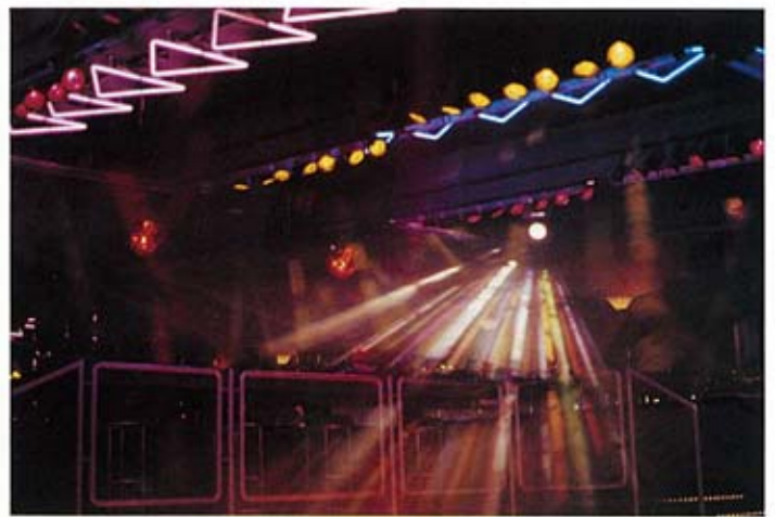
Effects lighting in The Barn comprises Raylights, Colour Sweeps and Fal's Florettes.
