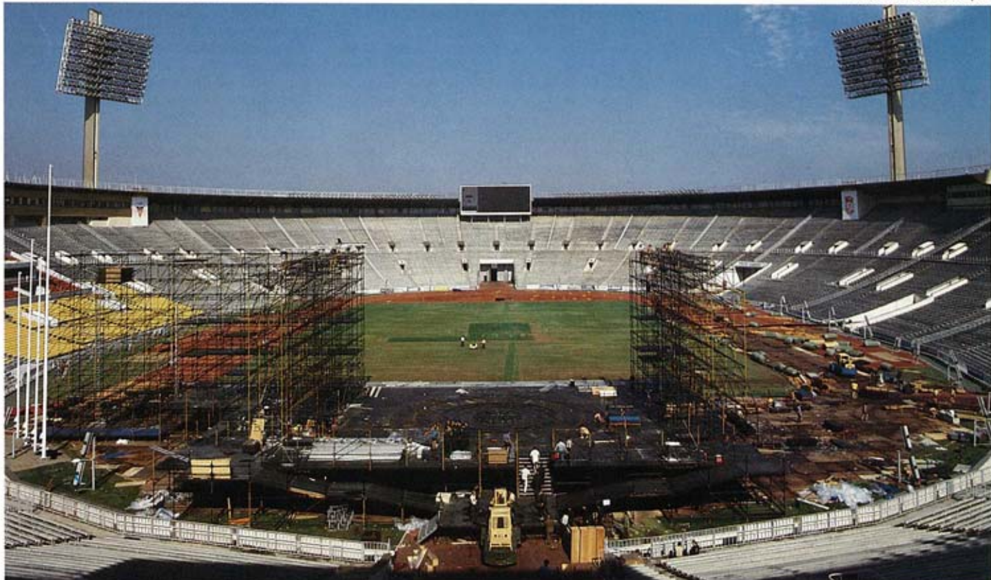
Set building and fit-up in progress at the Lenin Stadium, Moscow.
