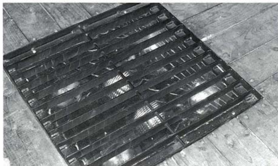
A close up of one of the stage floor lighting boxes, with section detail shown below.
