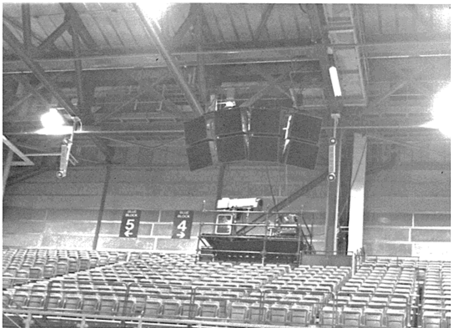
One of the Turbosound TMS-3 mini-clusters, part of the Quad system, with a follow spot station immediately below.
