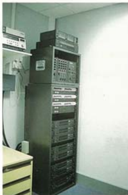
The sound rack (left) and the custom-zoning switch panel and microphone in the control areas at Big R.
