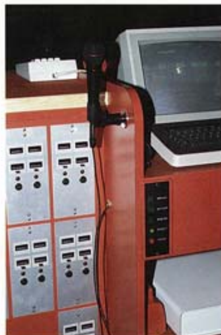
The sound rack (left) and the custom-zoning switch panel and microphone in the control areas at Big R.
