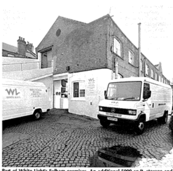
Part of White Light's Fulham premises. An additional 5000 sq.ft. storage and production area is based at Wandsworth.
