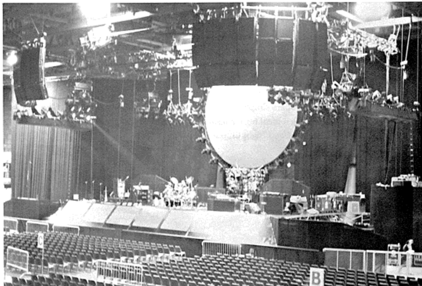
The main FOH PA (overhead) with in-fill cabinets behind black screens, stage left and right. Note height of stage (12') and circular projection screen (centre back).
