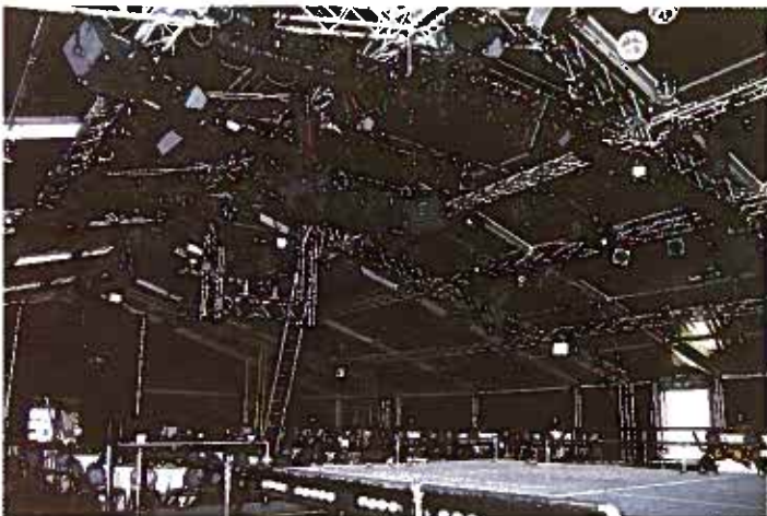
Currently on the road: Mushroom's major trussing scheme for Nationwide Anglia.
