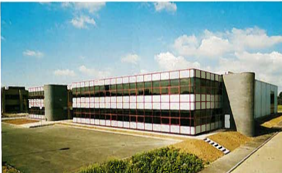
Strand Lighting's new HQ at Isleworth, Middlesex. One of the many new facilities is a comprehensively equipped studio/demonstration area.
