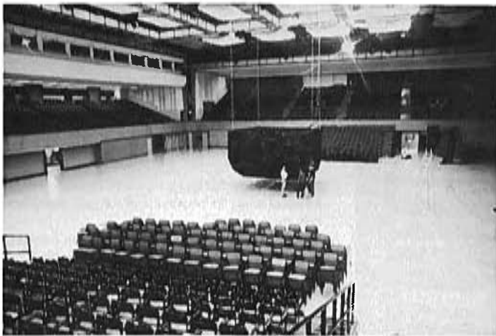
Members of Shuttlesound with cluster in the lowered position.
