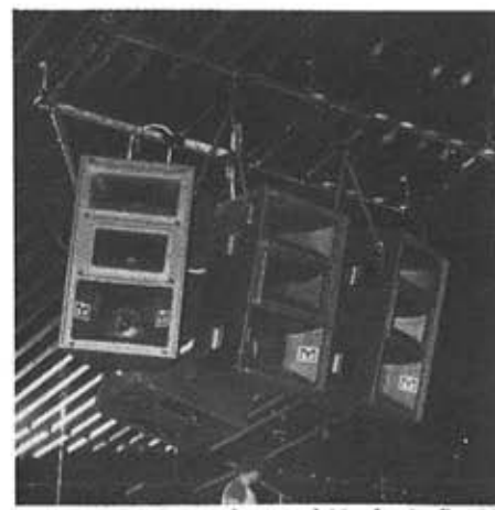
The left-side flown cluster of Martin Audio RS-1203D mid/high cabinets with VRS-800 at rear for stage audience coverage.
