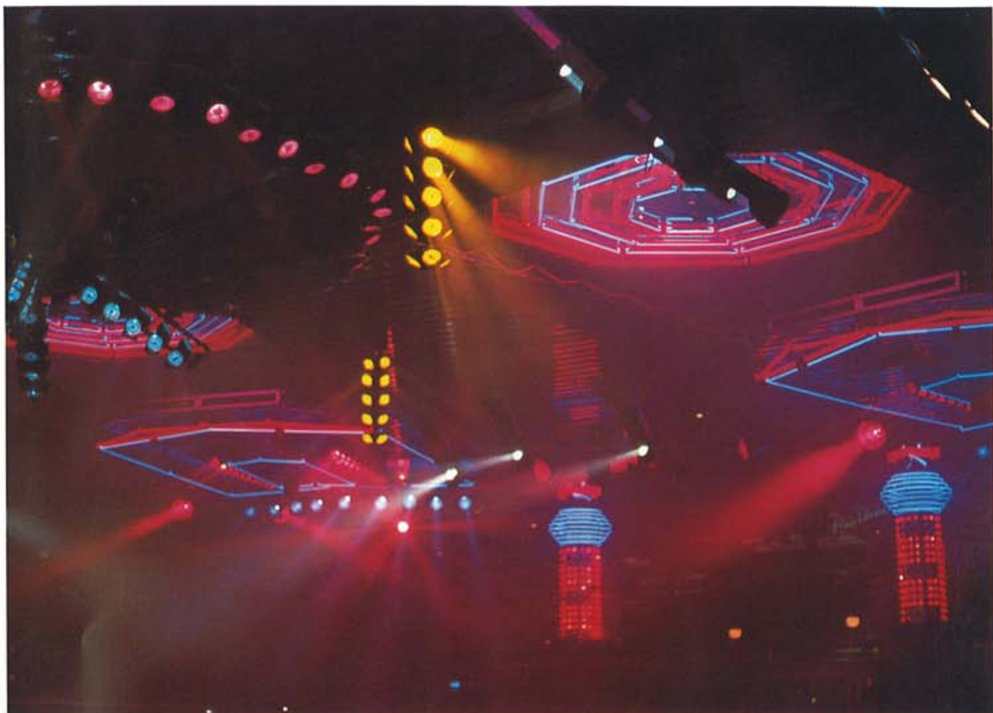
The covers are removed and the hidden telescopic units are ready to descend from the ceiling.
