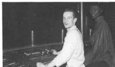
Le Palais' lighting controllers prepare to get the show on the road.
