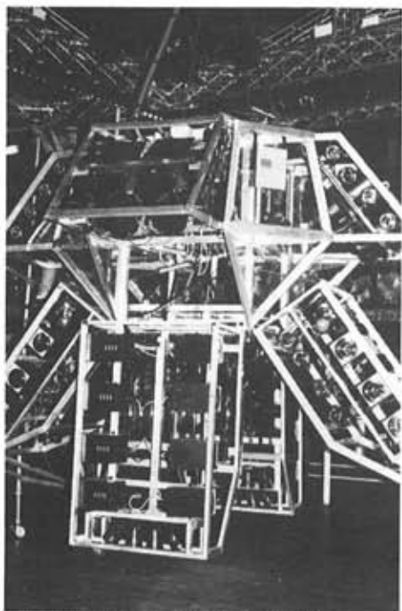
A close-up of the transformer centre-piece.
