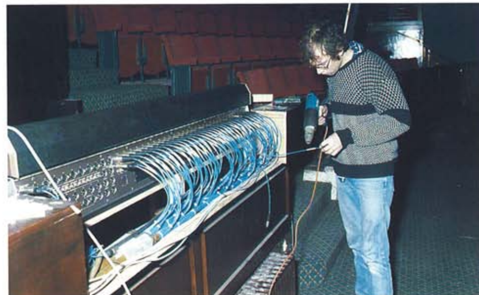
Part-completed mixing console cable form.
