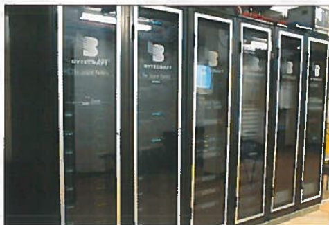
The rows of Bytecraft dimmers on one of the sound stages
