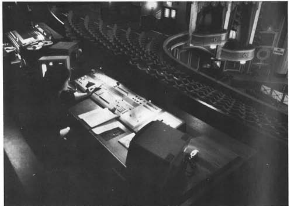
The Galaxy lighting control - and the sound desk - centre circle.
