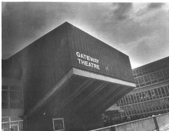
Chester's Gateway Theatre - the first Arri 'Image' control ordered outside London was installed here last month by Playlight.
