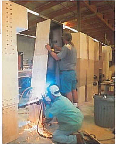
Above, the Titanic sign and inset, work in progress on the project
