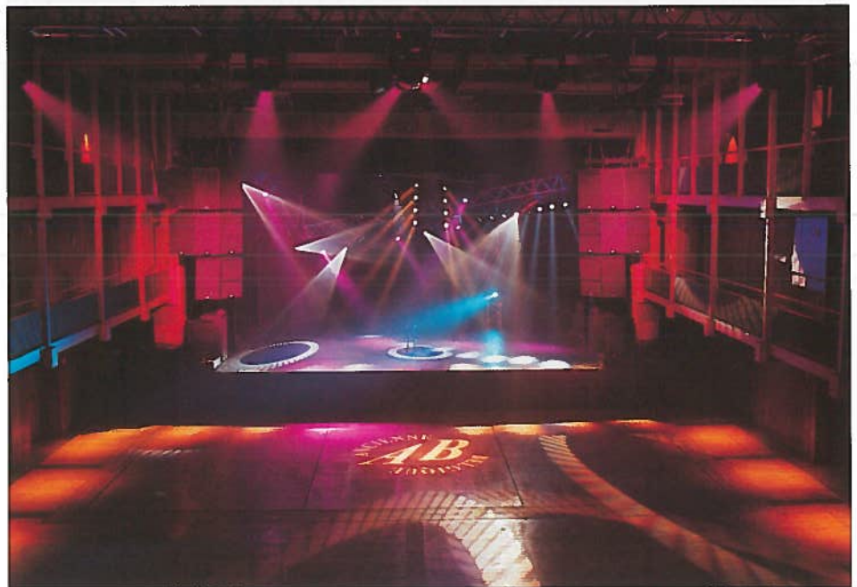
The main hall's new lighting rig in action - clusters of EAW speakers can be seen either side of stage.
