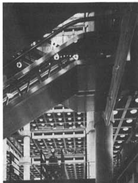
8,500 special lighting units were installed at the new Lloyds of London building.
