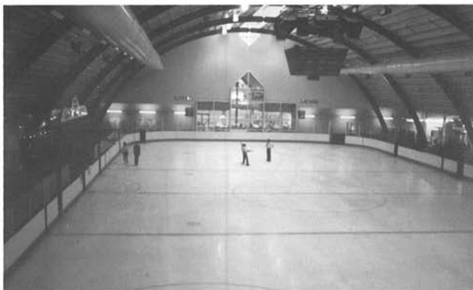
A general view of Slough Ice Arena. The FC100 priority paging horns are visible between each roof span on both sides of the rink. The unusual roof shape lent some positive characteristics to the reverberation.
