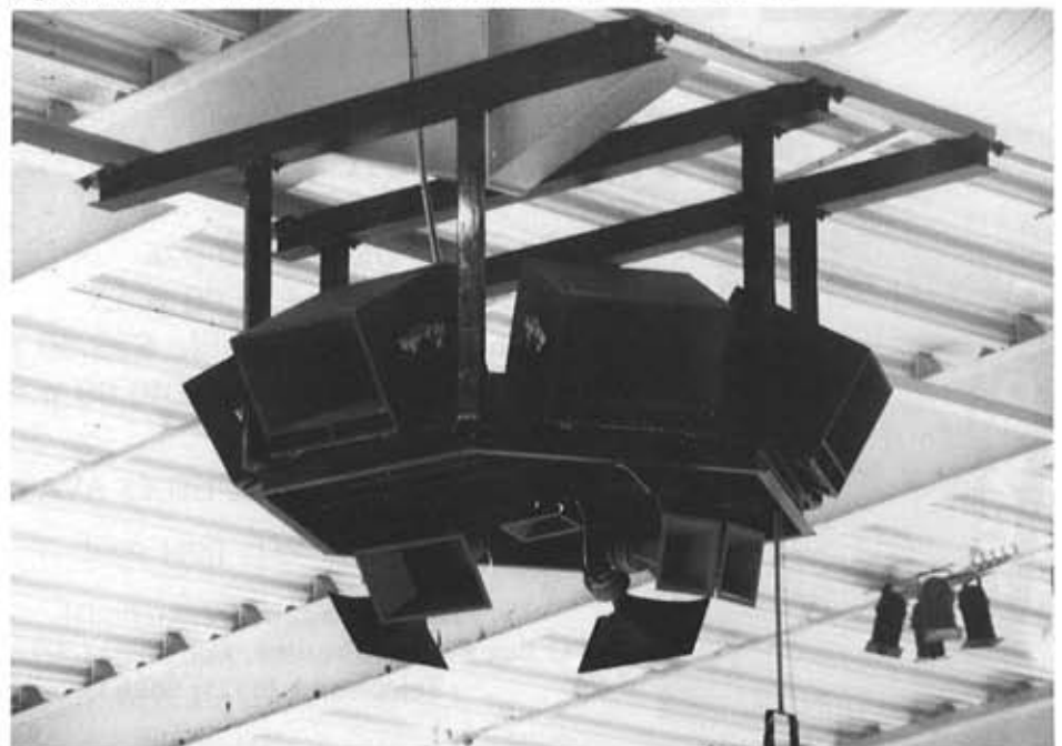
A close-up of one of the Telford Ice Rink loudspeaker clusters. The system can handle full-range music and also permit clearly audible announcements over crowd noise.
