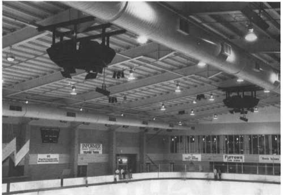
A general view of Telford Ice Rink showing location of the two loudspeaker clusters.
