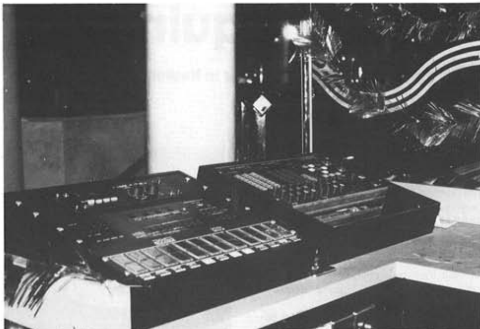
Control at the Millionaire with Light Processor with System Sensor and Arc Line control on the left, and Laser Systems' control on right.
