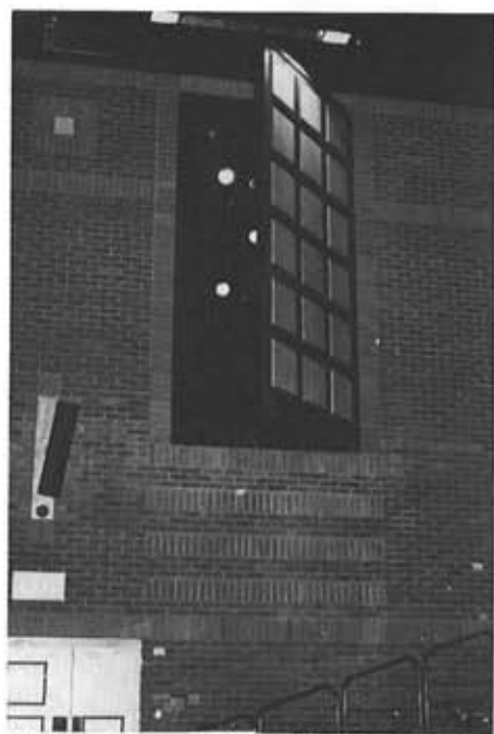
'Hide-away' front of house lighting positions at The Harlequin.
