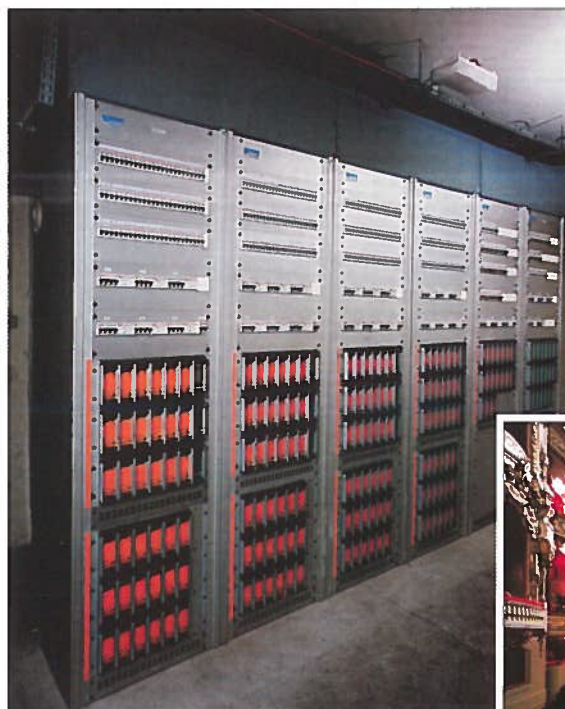
Above, HDD dimmer cabinets at the Opera de Nancy et de Lorraine (pictured right).
