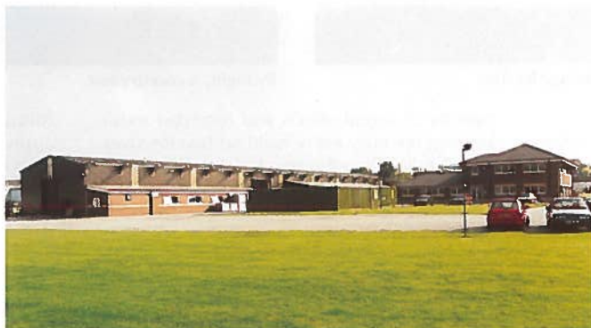
Acres of development space: the main warehouse will soon be expanded 'off picture' to the left.
