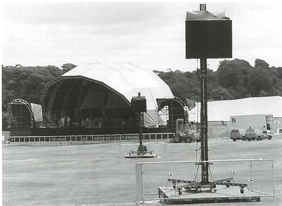
Paired EAW KF 850s on superlifts formed the delay towers at 55 and 105 metres from the stage.
