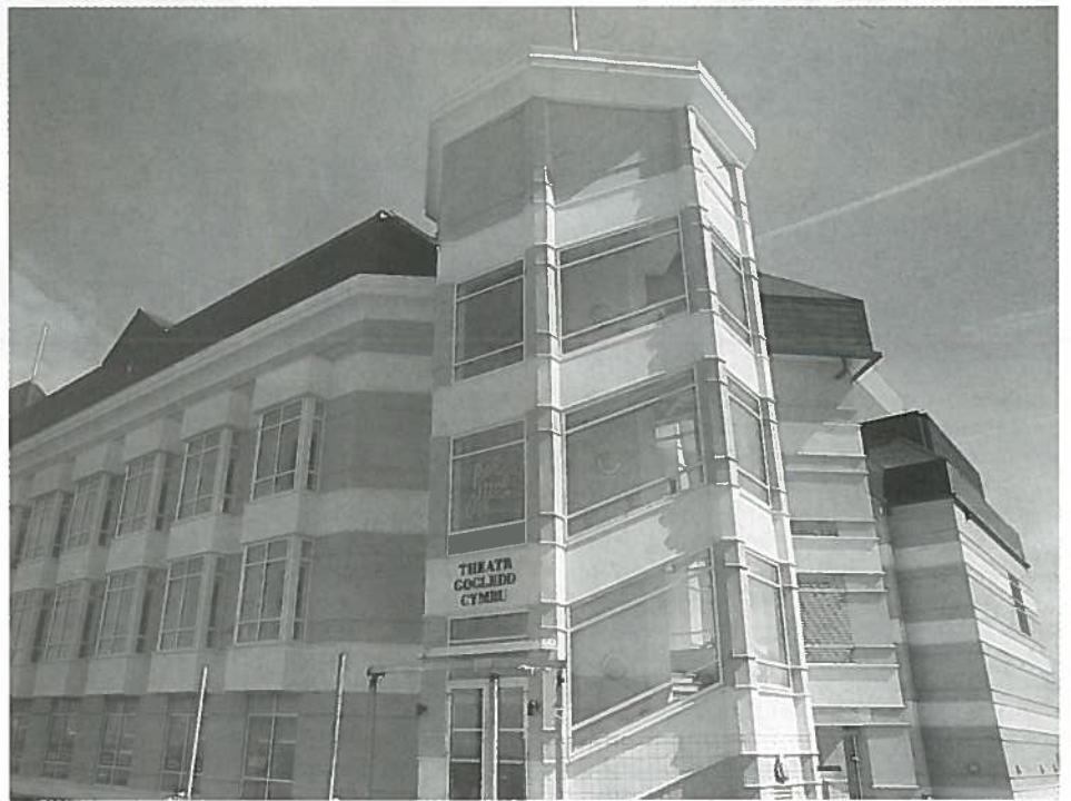
The latest addition to the Llandudno skyline is the modern facade of the North Wales Theatre.
