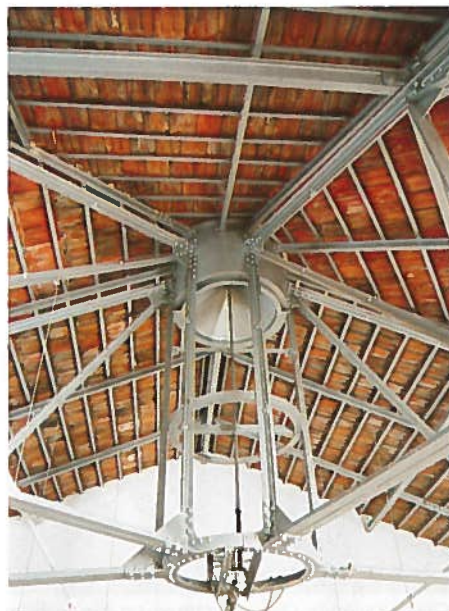
One of the refurbished Coliseu smoke lanterns.
